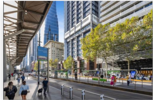
View from Southern Cross Rail Station – 120 Spencer Street
